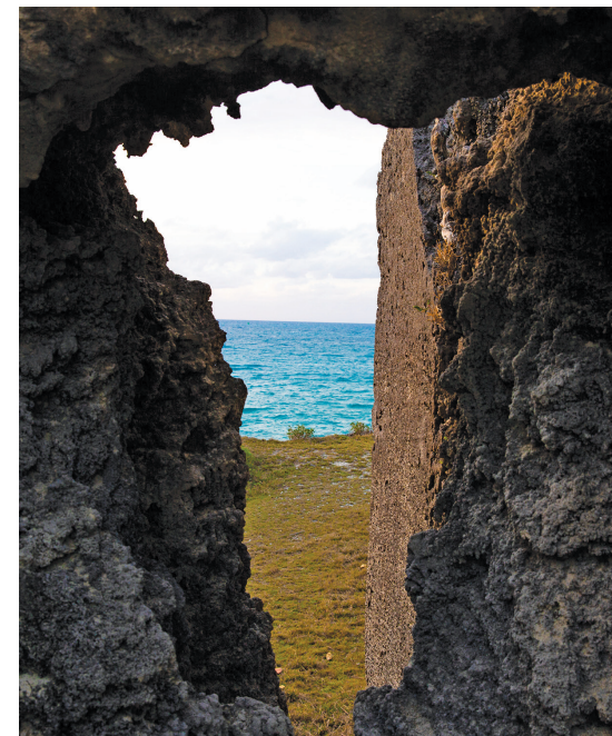
▲ Cuts such as this one at Shelly Bay were made in the limestone to allow for level train tracks.
