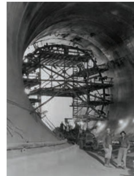
LEFT: A modern photo of Hoover Dam shows the recently completed bridge that bypasses the dam's roadway. ABOVE: A diversion tunnel is shown during the dam's construction in 1934.
