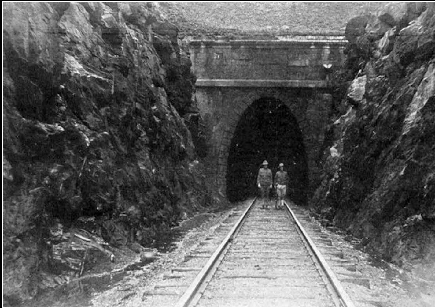
The west portal of the tunnel as it looked in 1917
