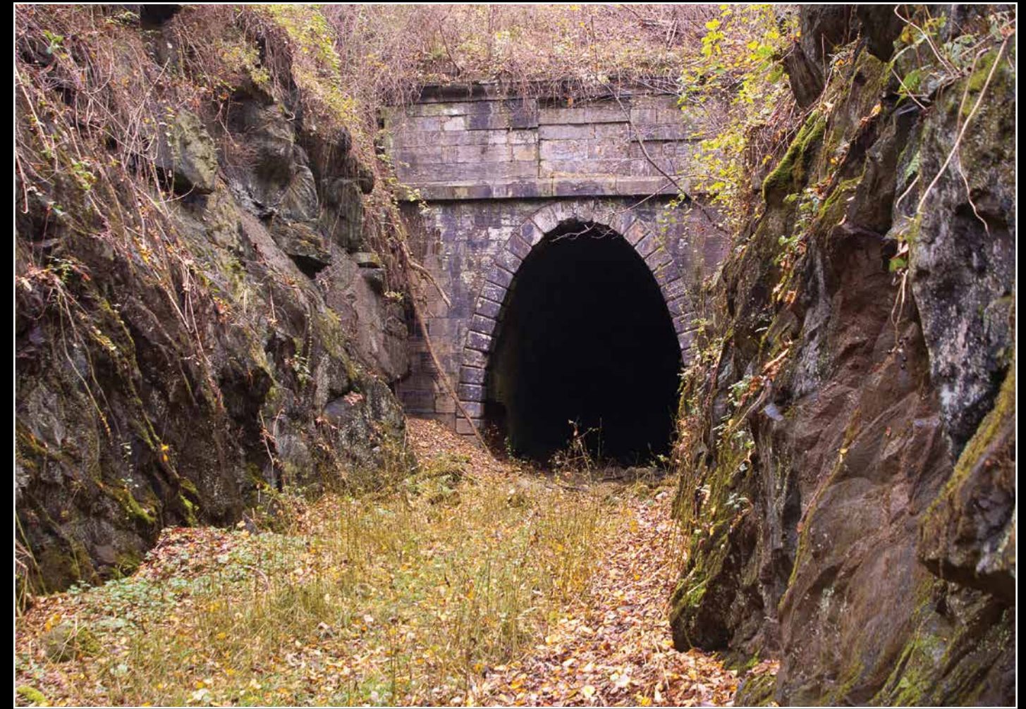
The west portal as it currently appears
