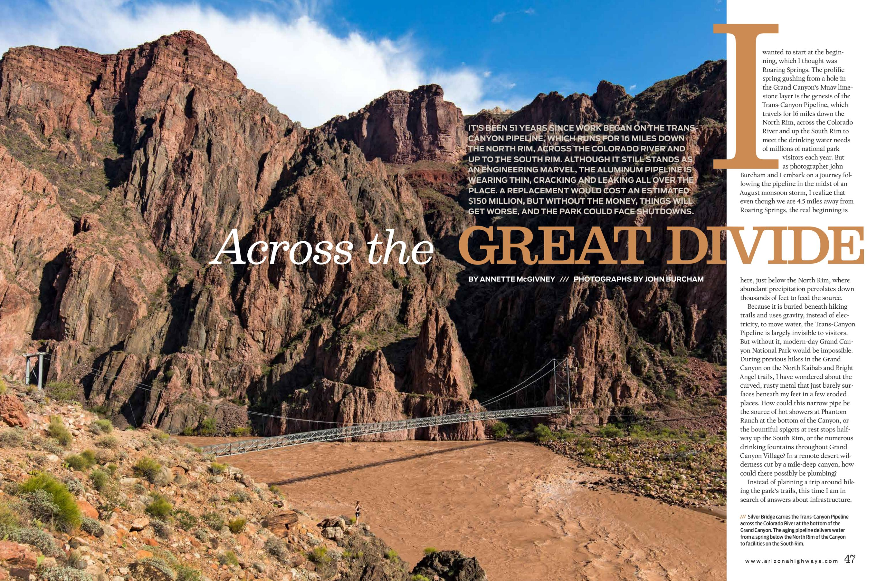
IT'S BEEN 51 YEARS SINCE WORK BEGAN ON THE TRANS-CANYON PIPELINE, WHICH RUNS FOR 16 MILES DOWN THE NORTH RIM, ACROSS THE COLORADO RIVER AND UP TO THE SOUTH RIM. ALTHOUGH IT STILL STANDS AS AN ENGINEERING MARVEL, THE ALUMINUM PIPELINE IS WEARING THIN, CRACKING AND LEAKING ALL OVER THE PLACE. A REPLACEMENT WOULD COST AN ESTIMATED \$150 MILLION, BUT WITHOUT THE MONEY, THINGS WILL GET WORSE, AND THE PARK COULD FACE SHUTDOWNS.
