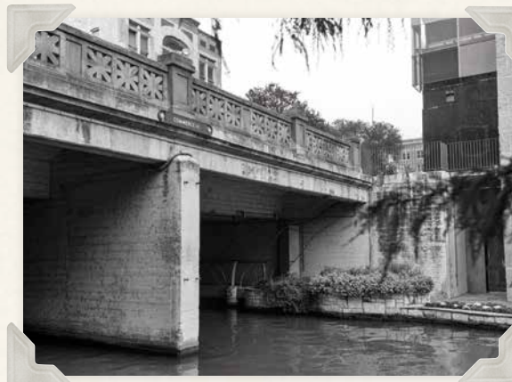
Commerce St. Bridge
