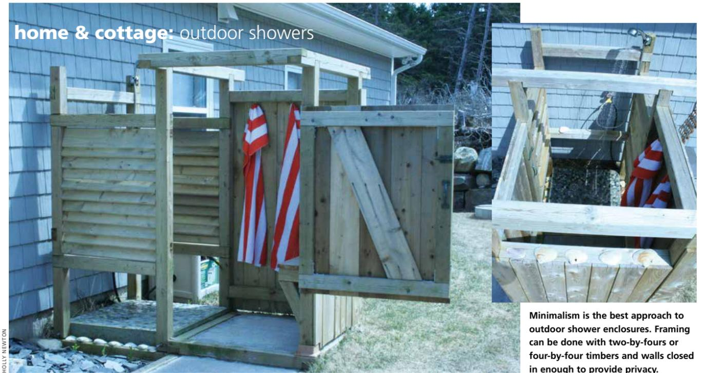
Minimalism is the best approach to outdoor shower enclosures. Framing can be done with two-by-fours or four-by-four timbers and walls closed in enough to provide privacy.
